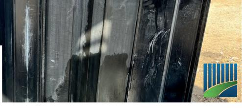
AIT Composites GWall® is a sheet pile system that utilizes a fully composites system including FRP sheeting and walers to provide a non-corrosive system that will not degrade for over 100 years.
