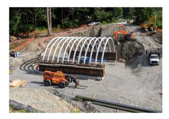
GArch™ is designed for short span bridges up to 80'.
